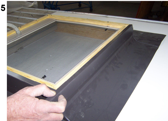
Install Counter Flashing on all Four Sides.
