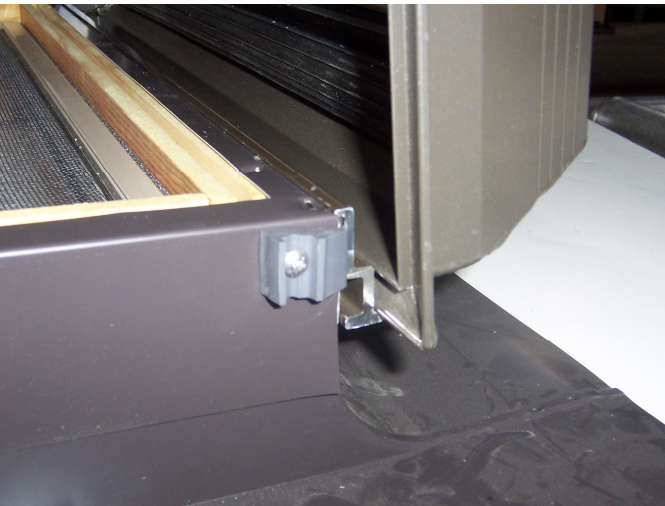
Stand top up at a 90° angle and install in hinge
