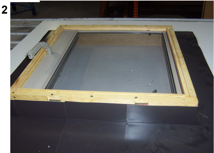
Remove rubber gasket and staples
